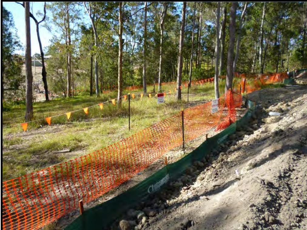
**FIGURE 15 – EXAMPLES OF VEGETATION PROTECTION FENCING**
